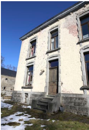
Figure 3. Building A: a case study in Mellier. Photo: Samuel Dubois.
