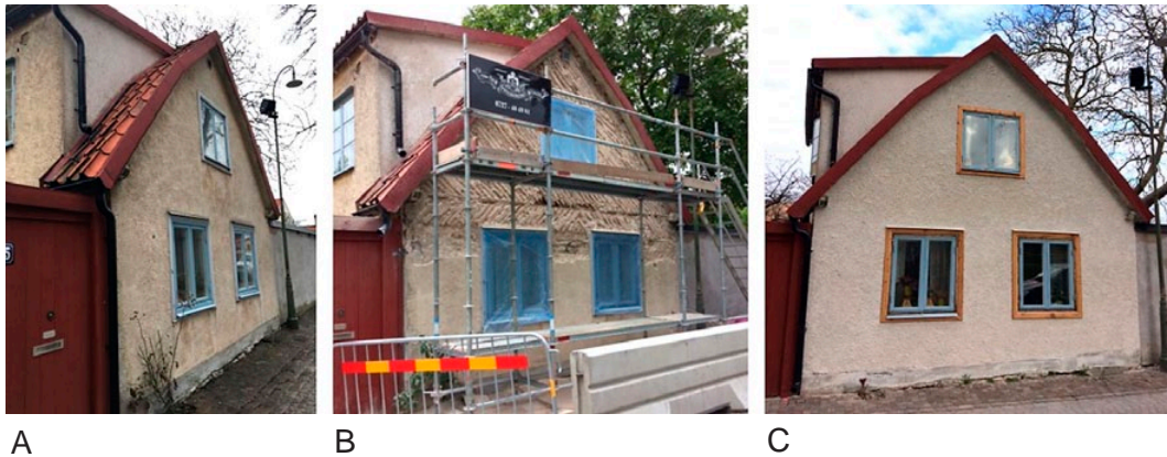
Figure 4. Detached historic single family house in Visby renovated with hemp-lime, A) Before renovation, B) During renovation, C) After renovation. Photos: Paulien Strandberg.
