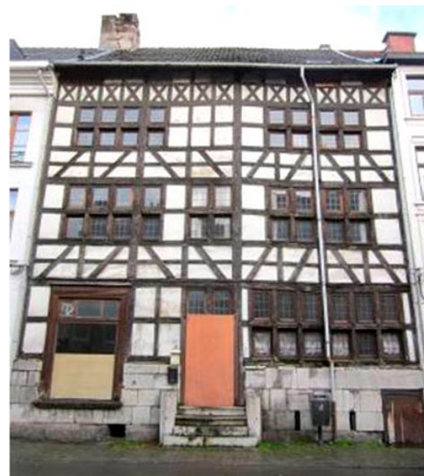
Figure 3. Main southern façade. Photo: AwaP.
