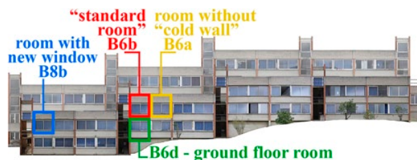
Figure 2. Position of the monitored rooms on the SW façade of the “Aquilone” building.
