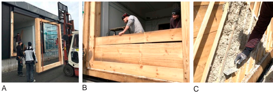
Figure 5. Construction of two full-scale test walls at Lund University, A) Construction of post-and-plank walls, B) Timber planks mounted between the posts, C) Application of hemp-lime on the post-and-plank wall. Photos: Paulien Strandberg.
