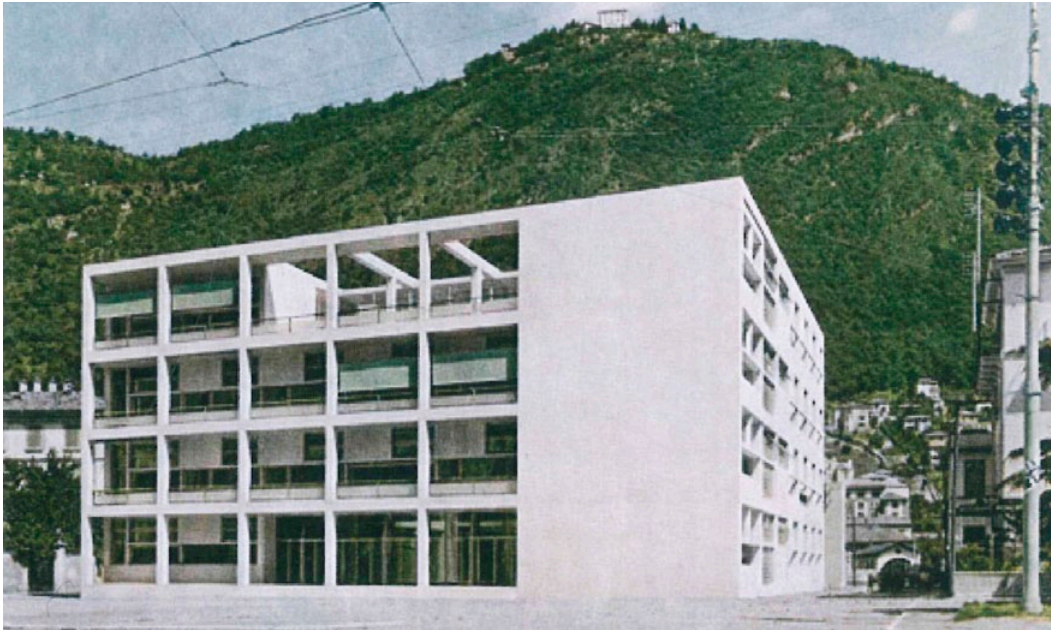
Figure 5. Old photo of the main façade on Piazza del Popolo, with the original green roller curtain system.
