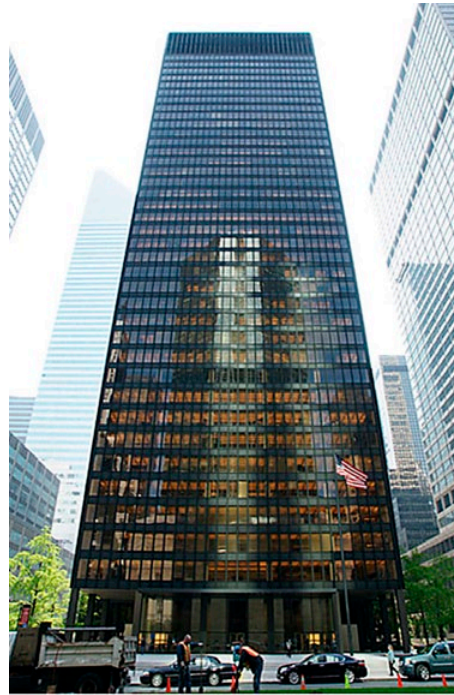
Figure 1. Example of mid-century Modernist curtain wall building (Seagram Building, New York, NY. Architects: Ludwig Mies van der Rohe and Philip Johnson). Photo: Wikipedia, open source.
